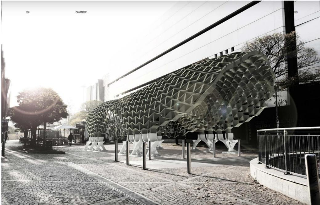
**Figure 2.45:** Pavilion: An architectural shell that cover an area of 18x6m made with polymers and metal supports. (Mirante 2015)
